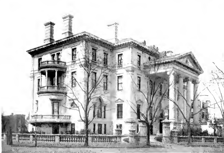
THE FEITER RESIDENCE.
